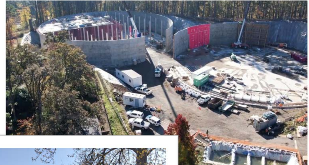
Construction of E. 40 th Storage Tanks
